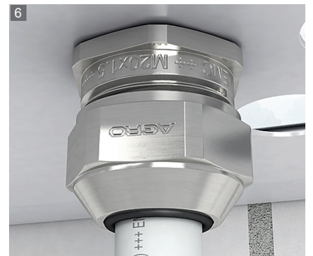
Tighten the cap to complete.
